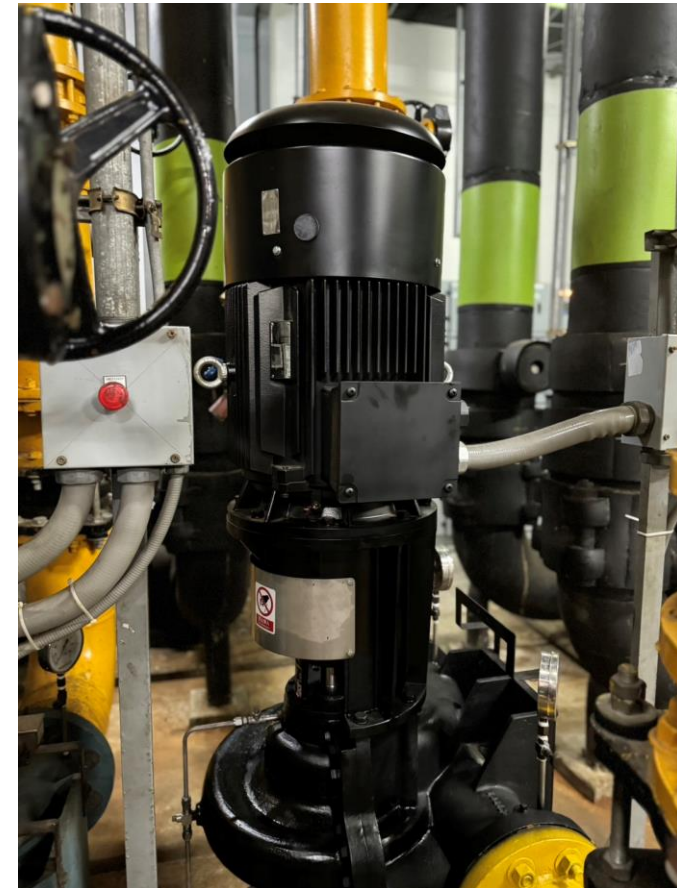
Replacement Water Pump
